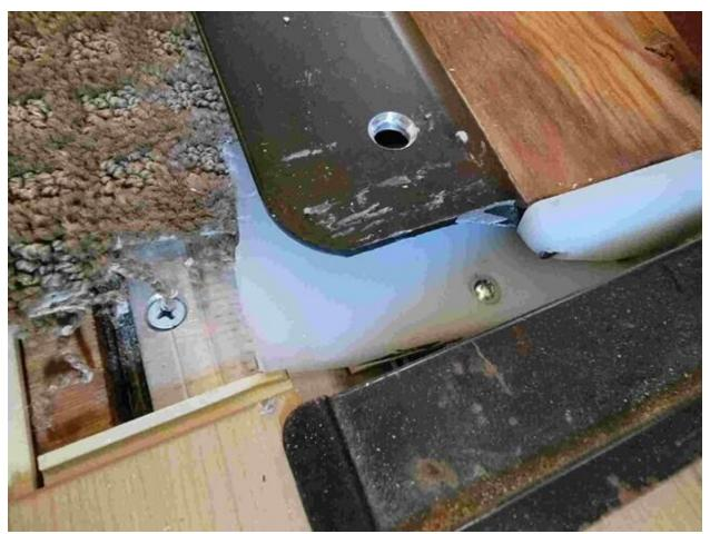
You will notice a hole drilled into the black alumimum edge of the slide. That is the access hole for screwing in the second screw.
