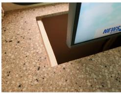
Countertop installed. I had to shave off a bit on the front side to fit around the round corner of kitchen sink cabinet. Picture above shows the small anti-rattle landing pads I had to install later.
