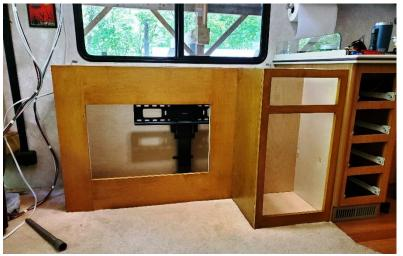
Cabinets/TV mount test fitting so I could cut the carpet out from under them and mount/shim TV Mount. Test fitting the TV mount showed me I needed 2" standoff from the wall to clear the window frame/ blind. Note the mounting piece on top and wiring bundles (power to left and video to the right) and the height of the cabinet relative to the window frame (it allows for a ½" thick countertop and a little extra space).
