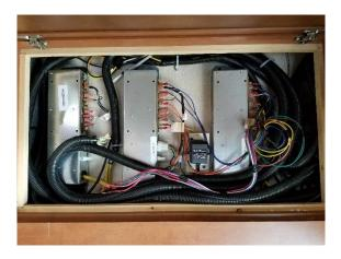
Connect the 120 volt, 20A, 12/2 w/g power wire and the loose bundle of wires for the A/C wire, freeze harness and single wires to the connections labeled R+, Cool Shed, Room, Freeze, Gen, B-, & Sig. Heat Shed is not used.
