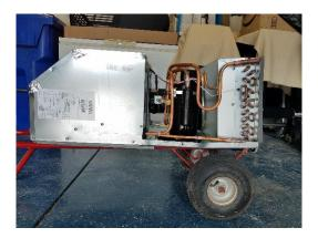
The new A/C controller – The factory installed A/C controller is usually a Coleman 8530C751 controller. Model numbers have changed over the years. We installed a Coleman 8630D5081.
