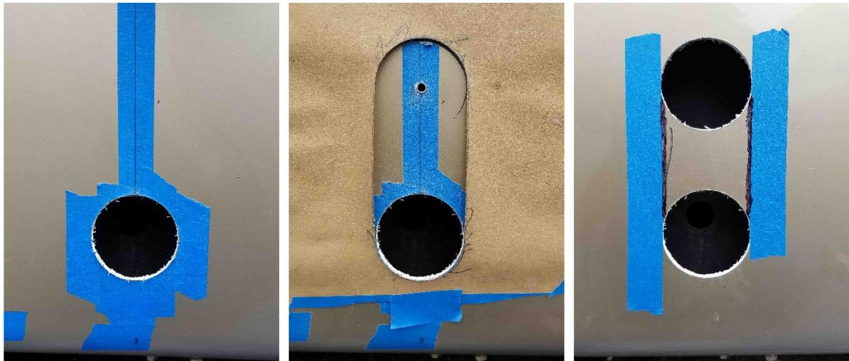
A little more trimming on the sides using a Dremel with a drum sanding head, insert the rubber grommet, insert the LED Fixture and finally insert the chrome ring.
