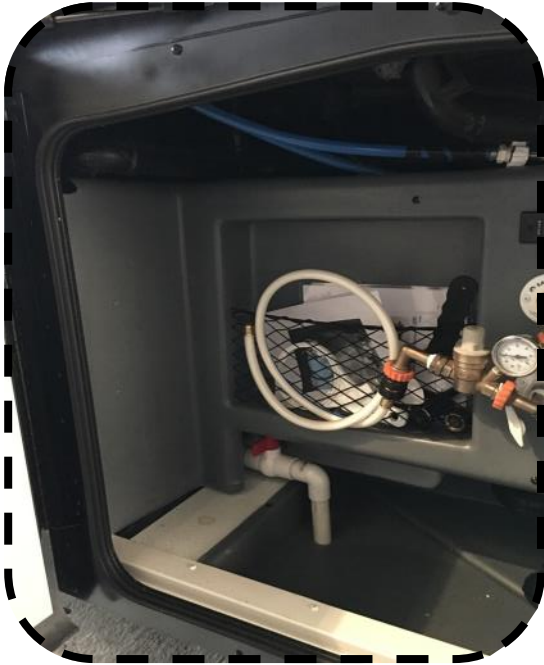
Bay after paper towel rack is removed
